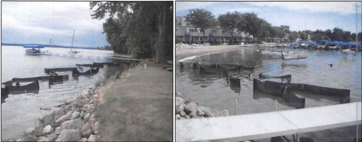
Figure 2: Protective enclosures were used to promote growth of vegetation by serving as wave breaks and wildlife deterrents.
